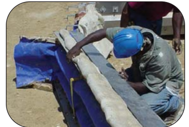
Thorburn's site team inspecting a section of a Flexi-Duct™ expansion joint before final assembly at a gas fired power plant in Australia
