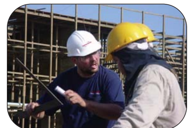
Thorburn's Site team providing expansion joint installation training in Tuxpan, Mexico
