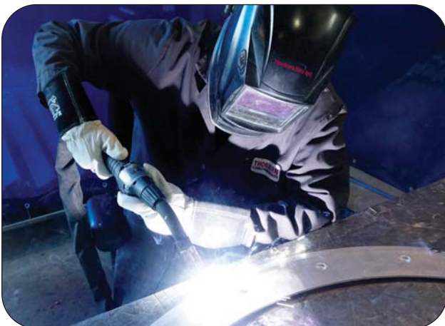
Thorburn's certified welder welding an aluminum 6061-T6 (SB-209) Flexi-Duct™ frame with ER 4043 AISI5 filler metal using Thorburn's certified ASME Section IX procedures
