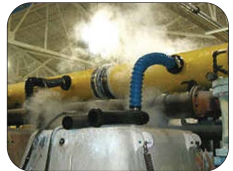
Thorburn Flexi-Duct™ BootFlex™ on a fume exhaust duct at a sulphuric acid plant
