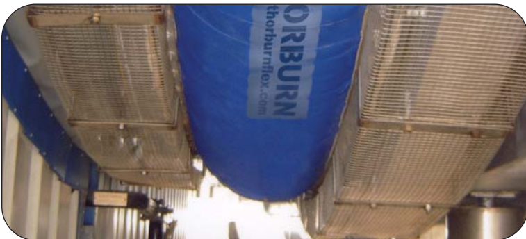
Mesh guard protection permits free convection and cooling of the expansion joint
