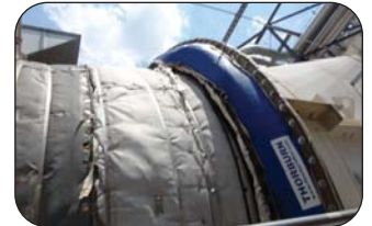
Thorburn Flexi-Duct™ CT outlet expansion joint
