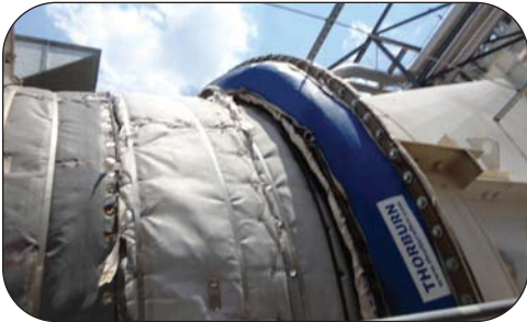
Thorburn installed a Flexi-Duct™ GTEJ-CC gas turbine exhaust expansion joint in Missouri USA
