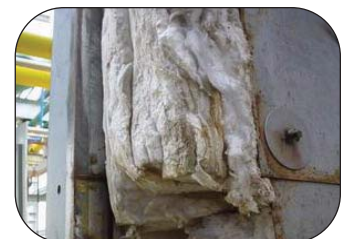
Pre-fabricated insulation pannels at a Dominican Republic HRSG/Gas turbine installation
