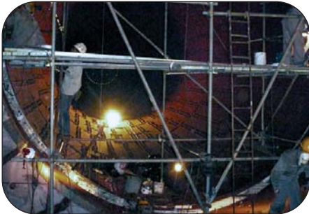
Gas turbine exhaust ductwork sloping downwards to the expansion joint
