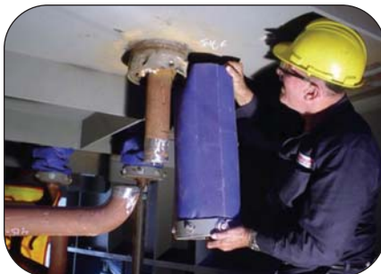
Installing a Flexi-Duct™ penetration seal
