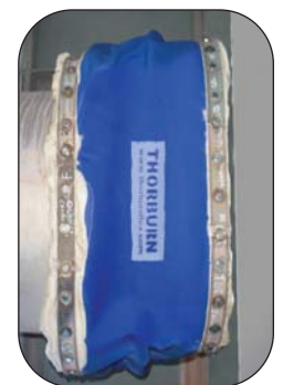
Thorburn Flexi-Duct™ high temperature 625°C penetration seal expansion joint on a single steam pipe system
