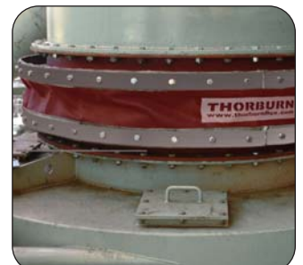
Thorburn Flexi-Duct™ TLFP GSM expansion joint for wet scrubber service
