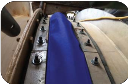
Flexi-Duct expansion joint with Shutter-Flex™ technology
