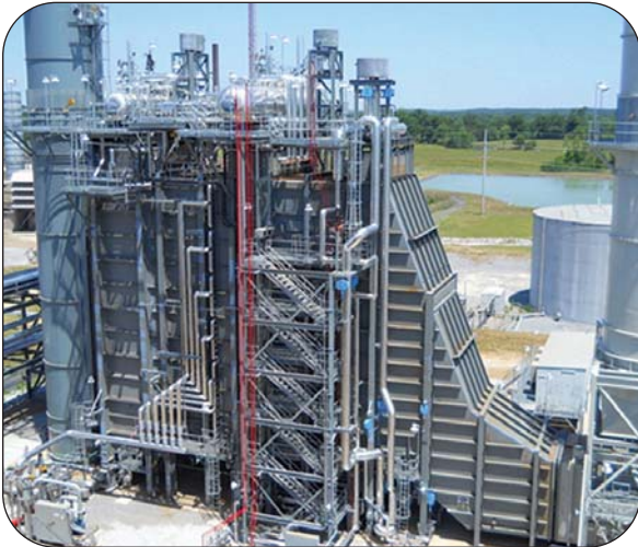
An HRSG system consists of four major components: the economizer, evaporator, superheater and water preheater. The HRSG recovers the waste heat available in the combustion turbine exhaust gas. The recovered heat is used to generate steam at high pressure and high temperature to run other turbines.
