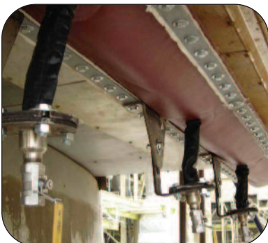
Flexi-Duct™ with M12 GSM and drainage system at a power plant in Alexandria, Egypt
