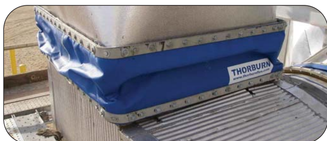
Thorburn's Composite Series FDC expansion joint GSMs are typically designed for ducting systems with temperatures above 204°C (400°F)
